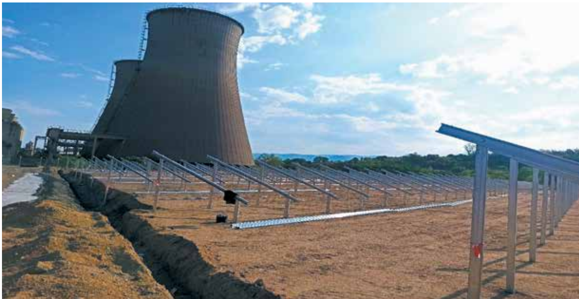
Installation of a 1 MW photovoltaic system and development of green-hydrogen infrastructure at this flagship project of the post-lignite era.
